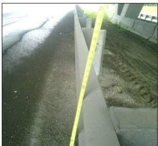
Left: Seward Highway – Missing block Right: Seward Highway – Horizontal tear
