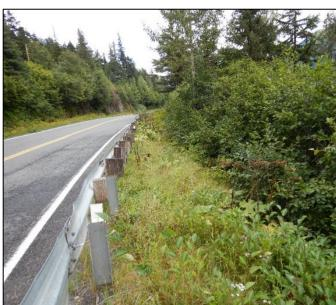
Left: Glenn Highway – Guardrail deflection and post separation Right: Glenn Highway – Guardrail failed due to height of rail
